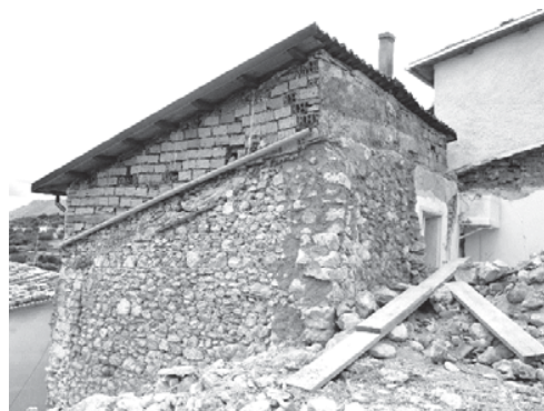
Fig. 3 Typical residential building
