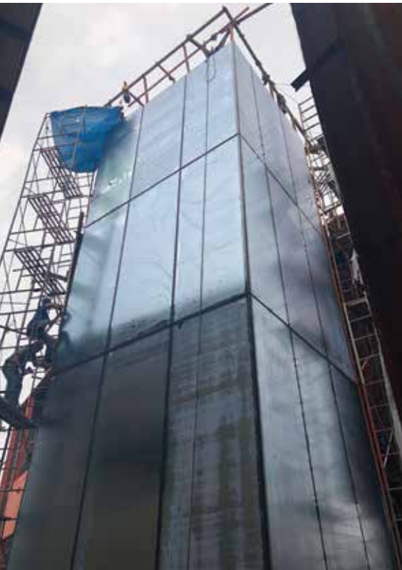
Figure 8.3. A mock-up installation at the Philippine Philco Façade test lab. © Angela Mejorin
