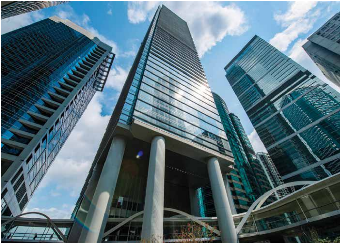
Figure 6.17. One Taikoo Place façade with connecting footbridge at podium level. © Swire Properties
