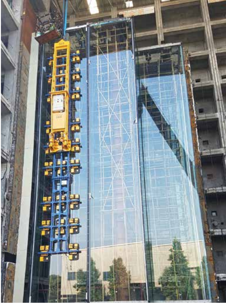
Figure 6.20. Performance mock-up of the podium façade. © Wong & Ouyang Architects
