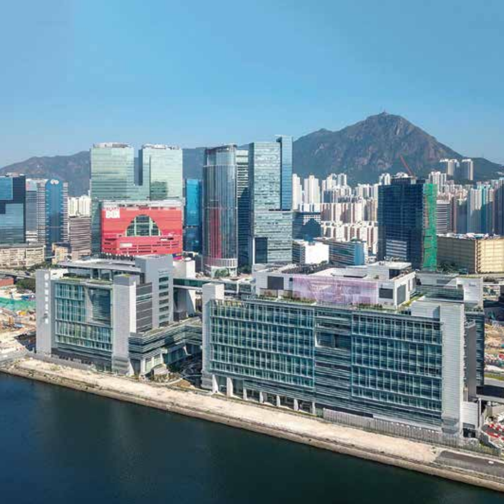
Figure 6.5. Hong Kong Children's Hospital, Hong Kong. © Wpcpey (cc by-sa)
