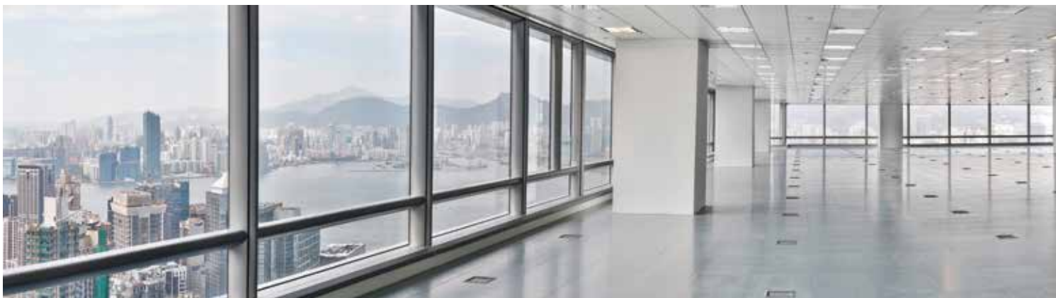
Figure 6.16. The view from the inside. The glazed curtain wall has modules measuring 2.4 meters high by 3 meters wide. © Swire Properties
