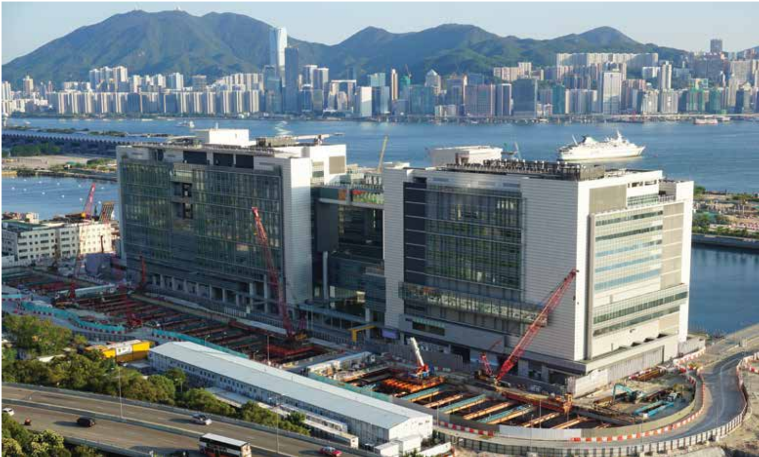
Figure 6.6. Alternate view of the Hong Kong Children's Hospital (HKCH) under construction. © Prosperity Horizons (cc by-sa)
