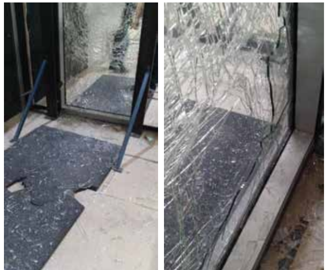
Figure 5.13. IMOC Windborne Debris Testing Procedure. The back pane completely shattered, but there was no penetration or dominant opening in the outer pane. © JML-Craft
