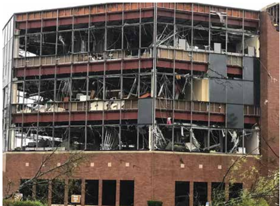
Figure 4.4. The damage to Florida's Panhandle by Hurricane Michael, 2018, was significant. © Jeff Gammons.
