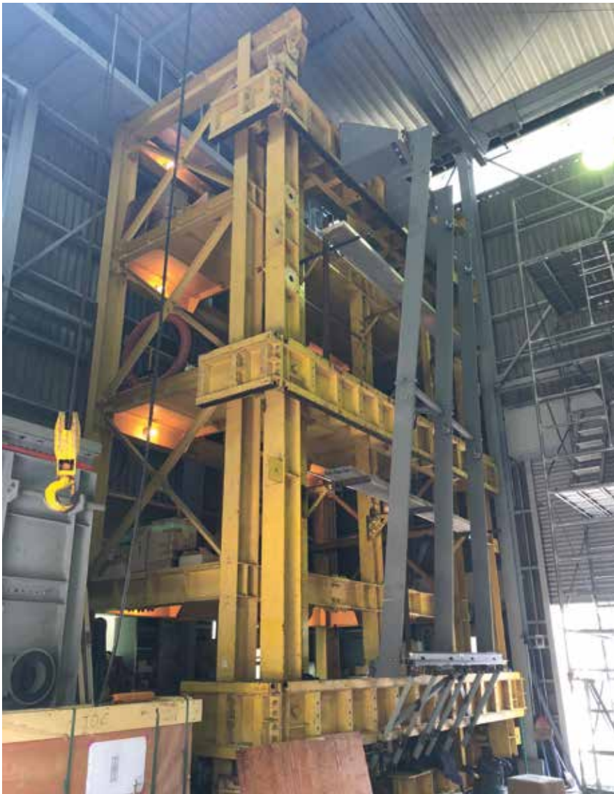
Figure 7.3. Façade mock-up installation for testing, General Building Research Corporation (GBRC). © Angela Mejorin
