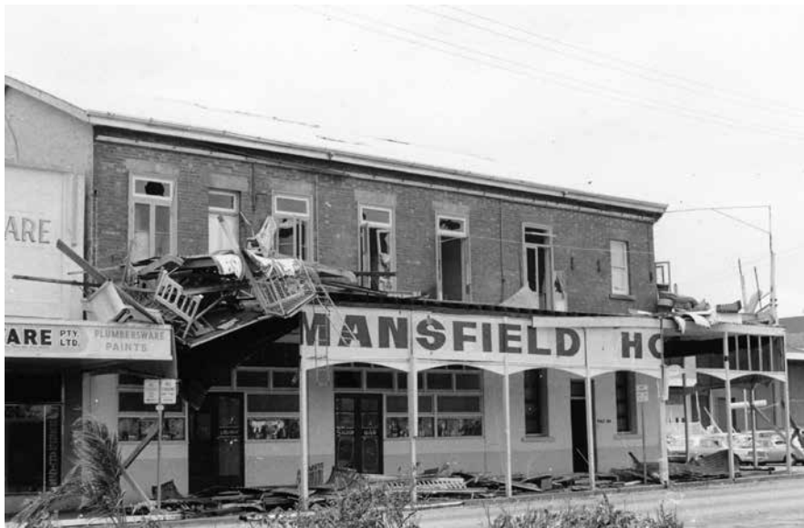
Figure 3.2. Damage to a hotel in Townsville, Queensland, after Cyclone Althea, 1971.
