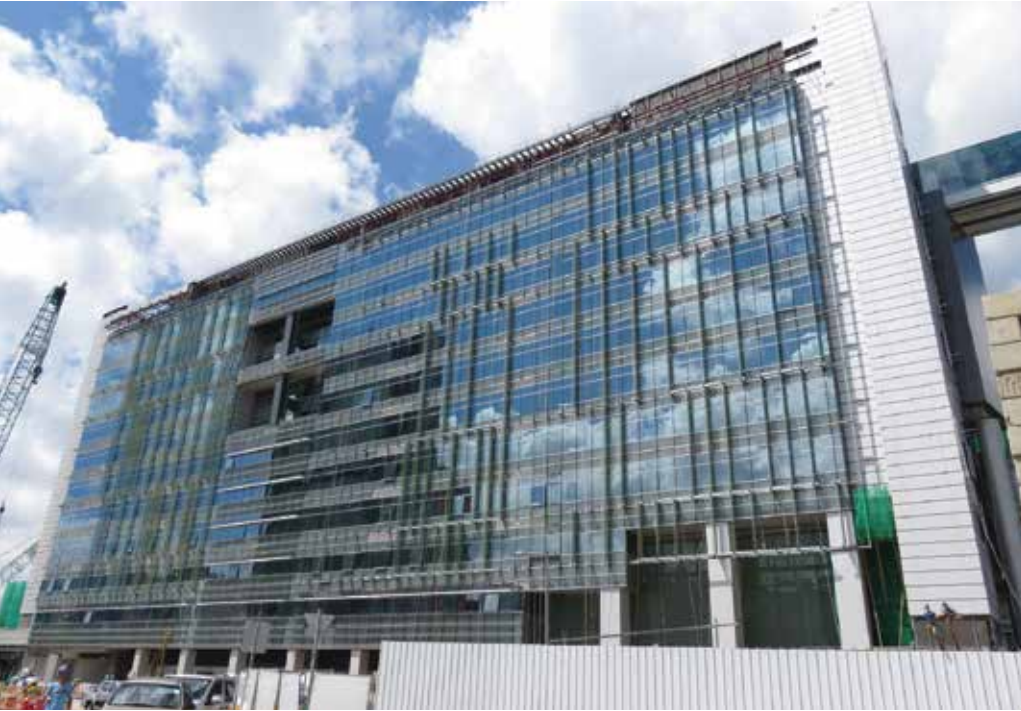
Figure 6.8. The curtain wall, as assembled on the Hong Kong Children's Hospital tower. © Meinhardt Façade Technology (HK)
