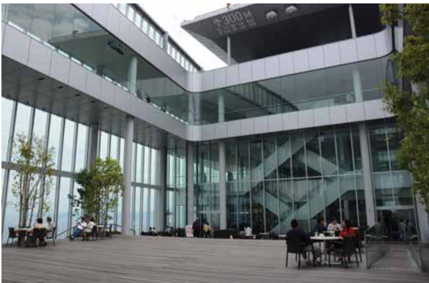
Figure 7.16. The partially enclosed observatory makes extensive use of glass treated for variations of wind pressure, based on location within or on the extended glass parapet. ©: Terri Meyer Boake
