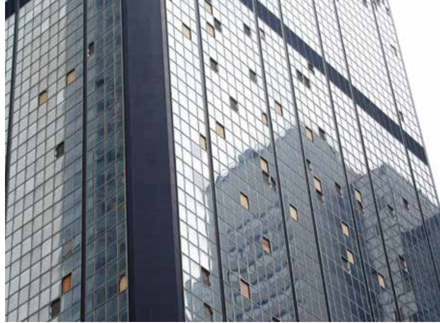
Figure 6.4. Typhoon York's winds shattered the curtain walls of several buildings in Wan Chai, Hong Kong, September 1999. © Joe Khoury/ALT Cladding
