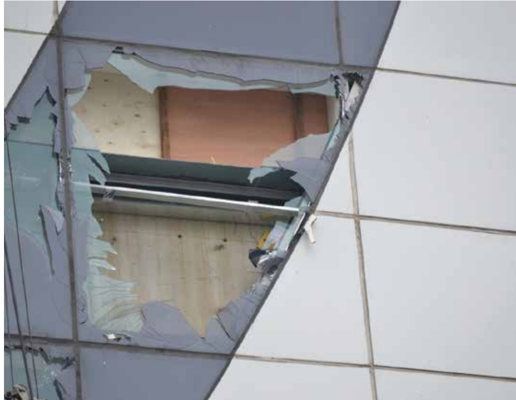
Figure 8.4. Typhoon Glenda, 2016, damaged glazed building envelopes in Manila. © Joe Khoury/ALT Cladding
