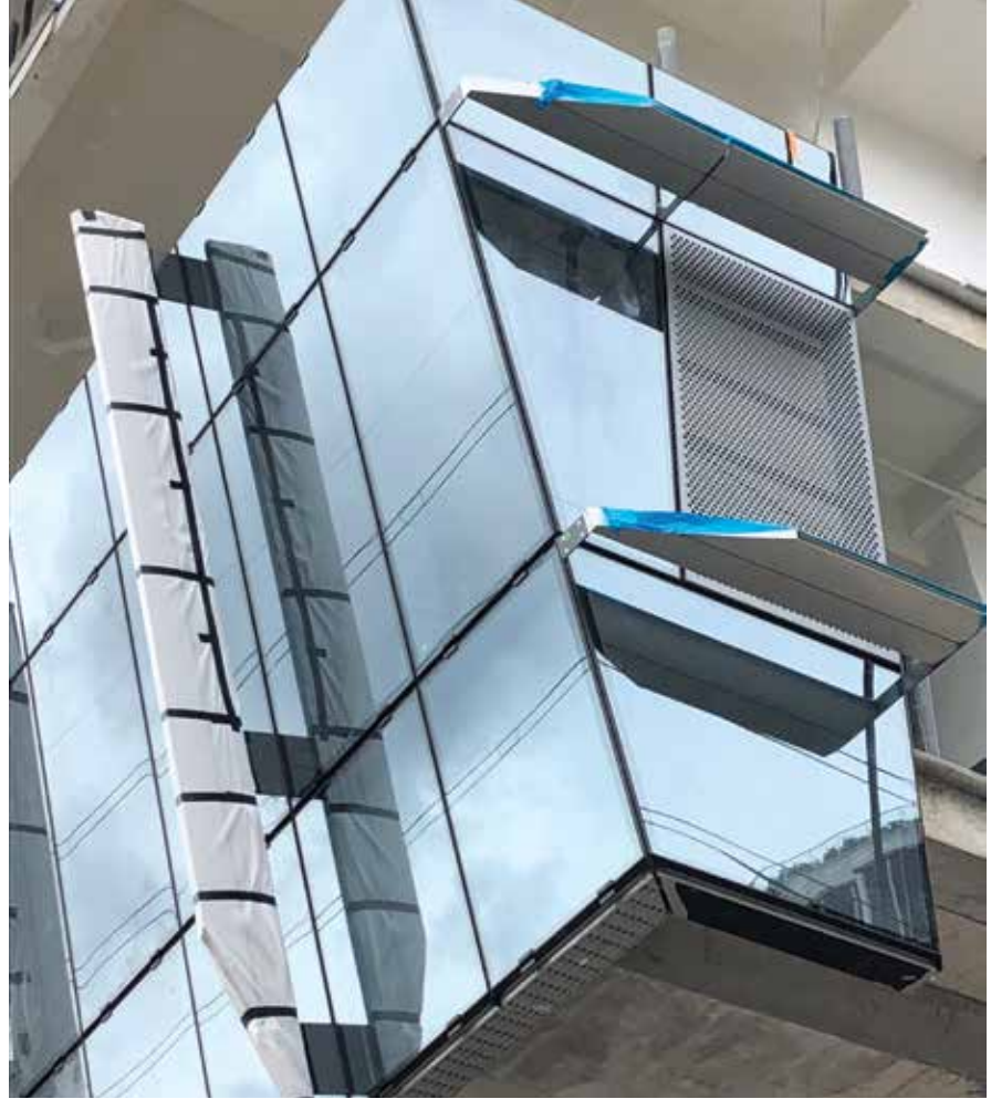
Figure 8.11. In-progress curtain wall installation. © SMEDD Corporation
