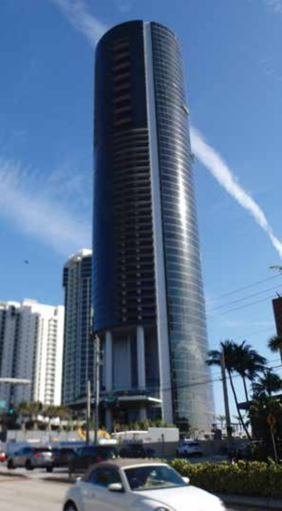
Figure 4.2. Porsche Design Tower, Miami (2017) extensively uses ionoplast interlayers in its façade. © Angela Mejorin
