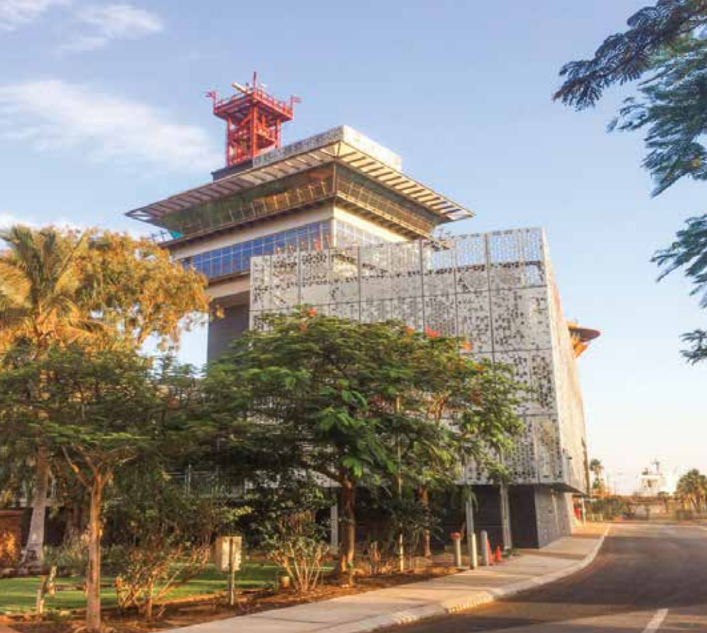
Figure 5.2. Integrated Marine Operations Centre (IMOC) tower, Port Hedland. © Pindan / JML-Craft.
