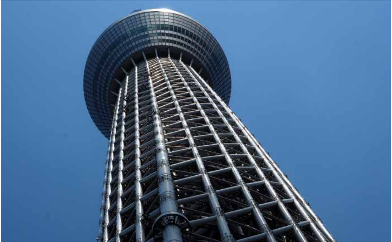
Figure 7.9 Tembo Deck curtain wall connection to the broadcast tower. © Andrew Currie (cc by-sa)
