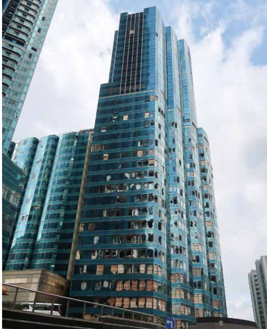
Figure 1.1. Damage to Two Harbourfront office tower in Hong Kong, after Typhoon Mangkhut, 2018. © Wpcep (cc by-sa)
