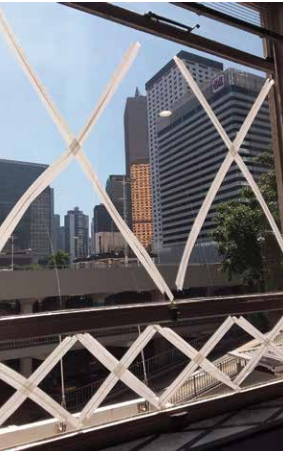
Figure 6.2. Hong Kong: Before the arrival of a typhoon, buildings use “X-tapes” to prevent injuries caused by glass failure that could occur due to wind pressure and windborne debris impact. © Msiuurjcos (cc by-sa)
