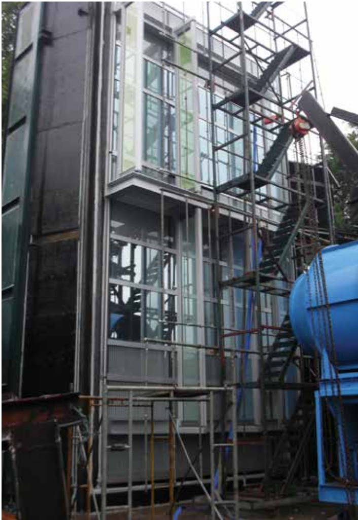
Figure 6.12. Performance mock-up for tower curtain wall. © Meinhardt Façade Technology (HK)
