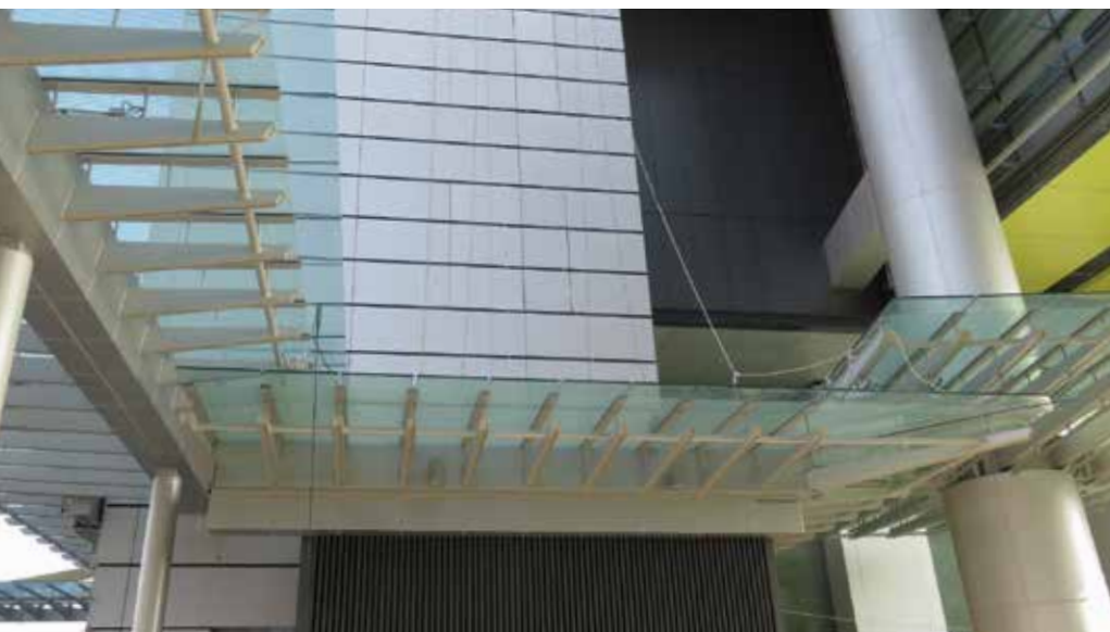
Figure 6.9. The canopy as constructed. © Meinhardt Façade Technology (HK)
