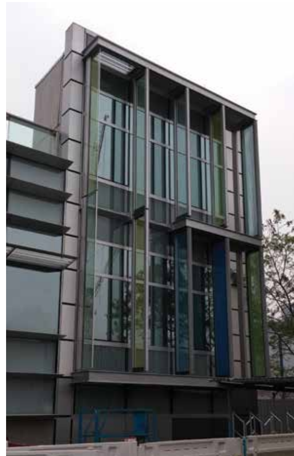
Figure 6.7. Full-scale visual mock-up of tower curtain wall. © Meinhardt Façade Technology (HK)
