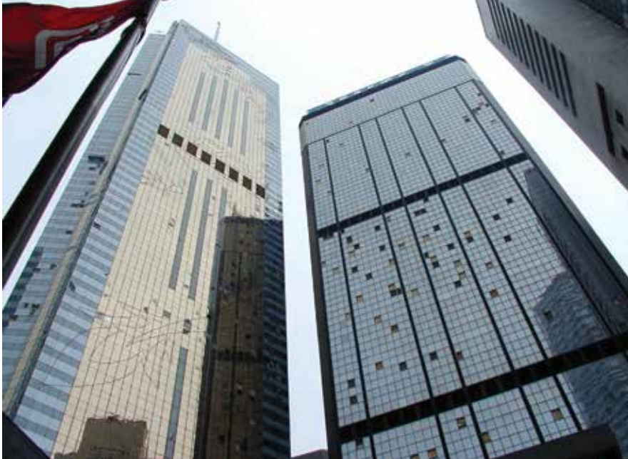
Figure 1.3. Typhoon York's winds shattered the curtain walls of several buildings in Wan Chai, Hong Kong, September 1999. © Joe Khoury / ALT Cladding
