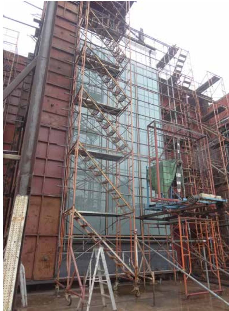
Figure 6.13. Performance mock-up for glass wall (alternate view). © Meinhardt Façade Technology (HK)
