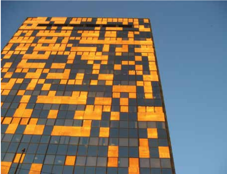
Figure 2.2. Plywood repair panels were visible on the Colonial Bank building, Miami, after Hurricane Wilma, 2005. © Jordan Fischer (cc by-sa)
