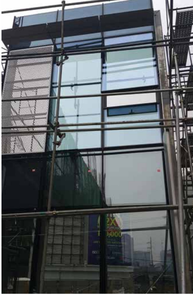
Figure 8.12. Façade mock-up. © B.L. Gavino Façade Design Consultancy
