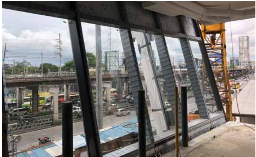
Figure 8.9 : Inclined curtain wall installation. © SMEDD Corporation
