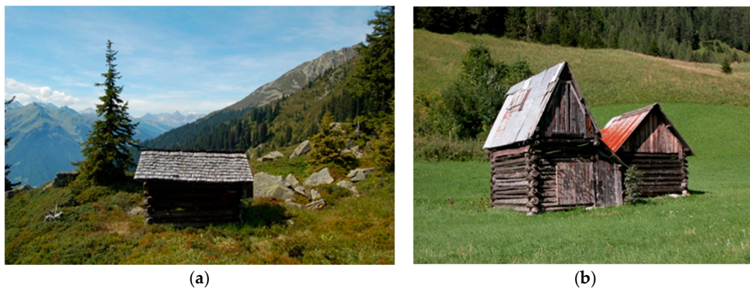
Figure 3. These “Heubarge” (“baita”, “barco”) (type 2C) mainly occur in the Alps to serve for hay storage: (a) traditional haylofts, (b) block huts (photos: left: Peter Strasser, right: Viviana Ferrario).
