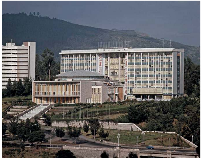
Figure 6: Anonymous, Africa Hall in Addis Ababa, 1963. Source: courtesy of Archivio Privato Mezzedimi (Italy, Rome).
