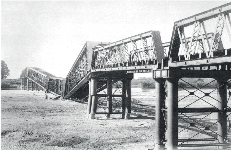
Images 8 - 9: Photographs of the effects of the Nōbi earthquake Source: John Milne and Ogawa Kazumasa, The Great Earthquake of Japan (1892)
