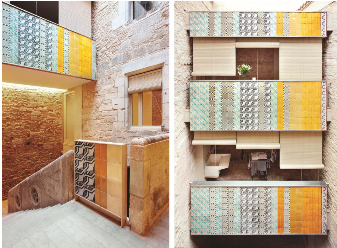
Fig. 9 - Bosch.Capdeferro architecture, Casa collage. Reuse of reclaimed ceramic pieces, mosaics and stones in a refurbishment: views of the inner patio. Girona, Spain, 2009. Credits: José Hevia.
