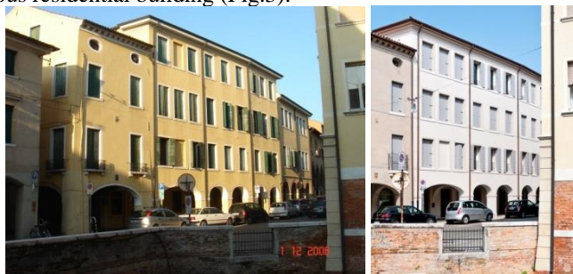
Fig. 3 General view of the building a) before and b) after the intervention.
