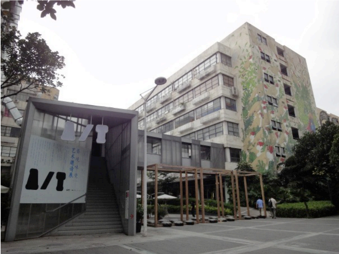
Figure 17. Section of the webbed corridor system (September 2012) – point n. 13 in Figure 9
