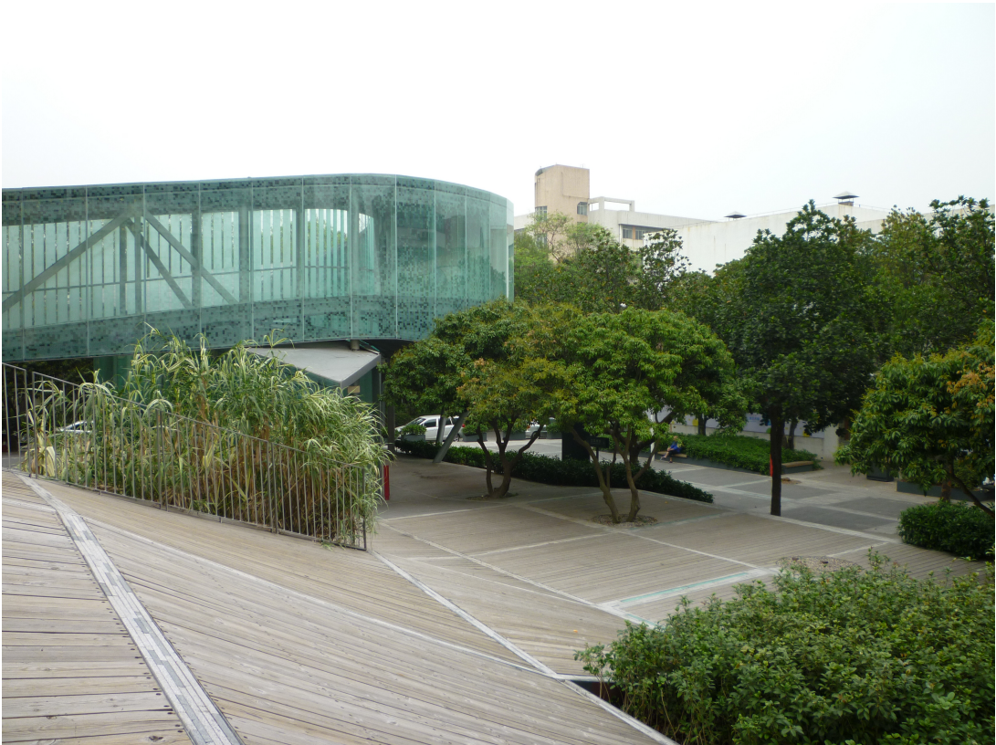
Figure 18. A5 building spiral stairs (September 2012) - point n. 16 in Figure 9
