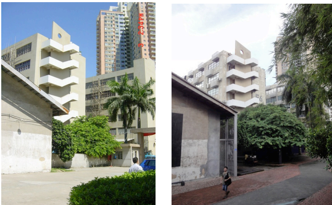
Figure 10. OCAT and E6 building – on the left, picture before the renovation (courtesy of URB, July 2003), on the right, picture after the renovation (September 2012) – points 3 and 7 in Figure 9
