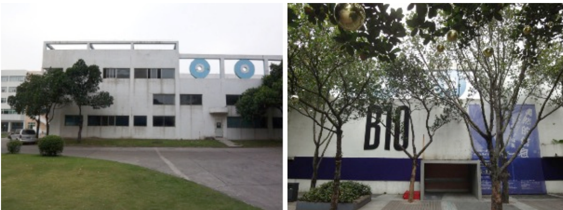
Figure 15. B10 renovation – on the left picture before the renovation (courtesy of URB, November 2007), on the right pictures after the renovation (September 2012)
