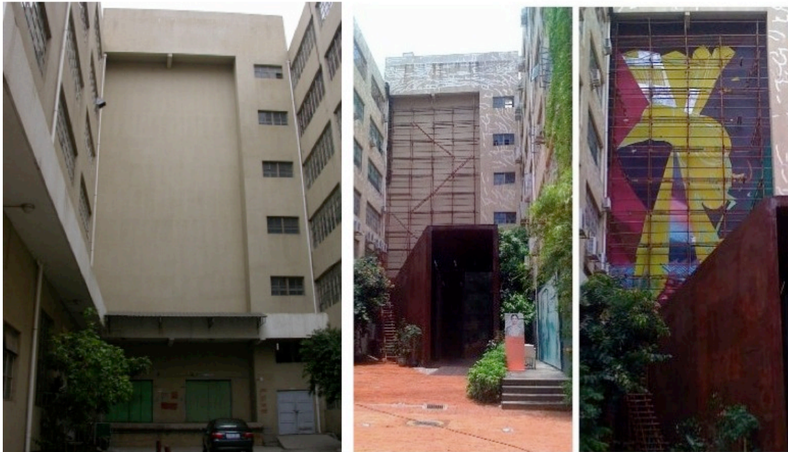
Figure 12. E6 building façades renovation – on the left picture before the renovation (courtesy of URB, March 2004), on the right pictures after the renovation (June 2011) – point n. 3 in Figure 9
