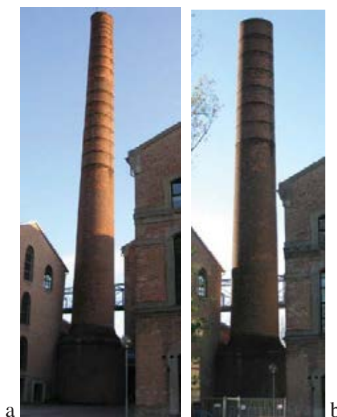
Figure 1: Masonry chimney in Ferrara before (a) and after (b) shortening [5].
