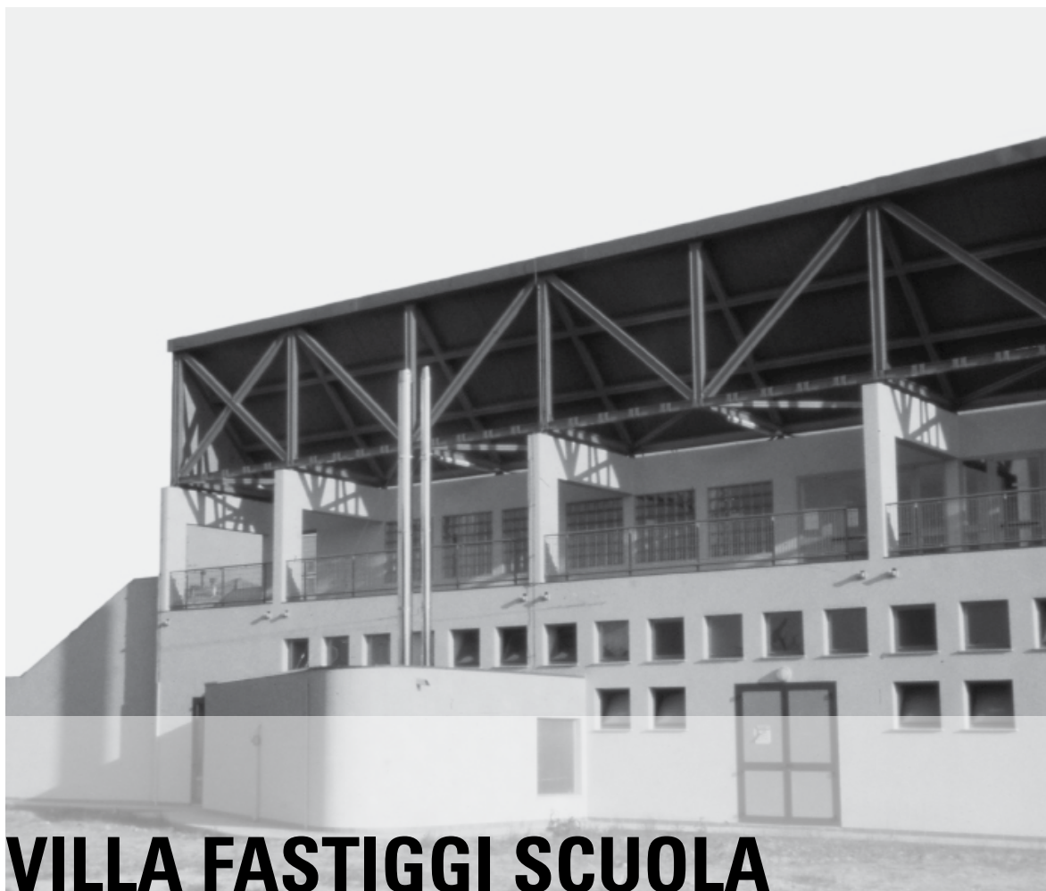
View of the west end with the gymnasium building and the balcony for the stand
