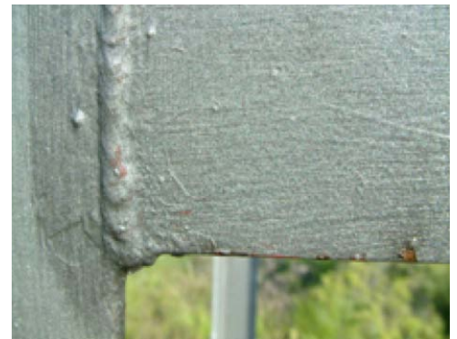
A weld seam from 1935 without any rust
