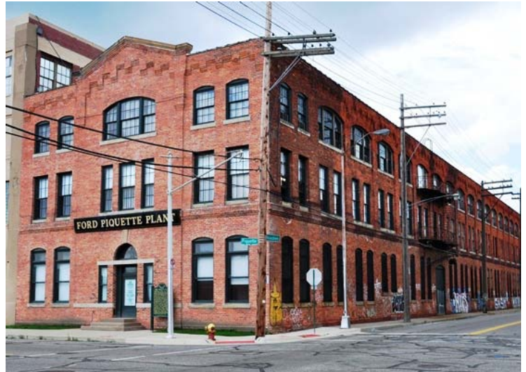
Ford Motor Company Piquette Avenue Plant, Detroit, is not considered significant for its structure, an unremarkable nineteenth century mill design selected primarily for open space hand-manufacturing. The tools and equipment it contained were equally unremarkable, designed for nearly any type of industrial production. Photo: Detroit Historic Building Archive
