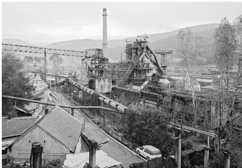
The giant Resita steel mill in Rumania, partly shut down in 2002. The last blast furnace is the fifth generation on the same site, with three Cowper preheating stoves, raw materials silos and plumbing all declared historical monuments since 2003. See Oana Țiganea's report on conserving Communist heavy industry. Photo: Viktor Mácha
