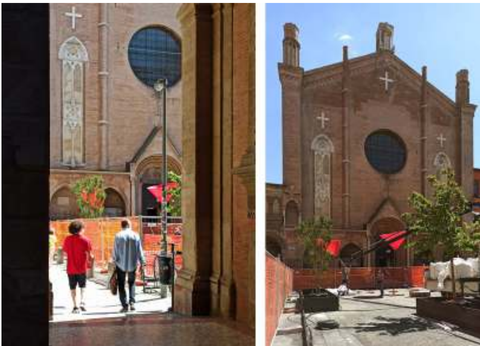
Figure 5: The “Green Please 2.0” project under construction, June 2020. (Source: ROCK Project, 2020 [8]. )
