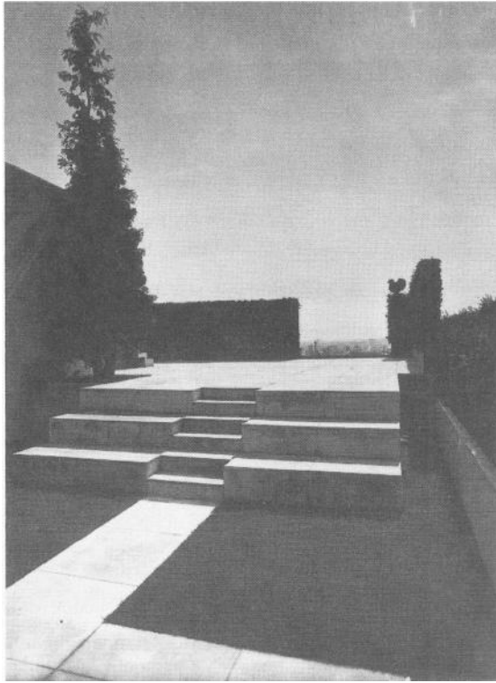
17 Penthouse for Charles de Beistegui, roof garden (photo Marius Gravot, FLC L2(5)21 ©FLC-ADAGP).
