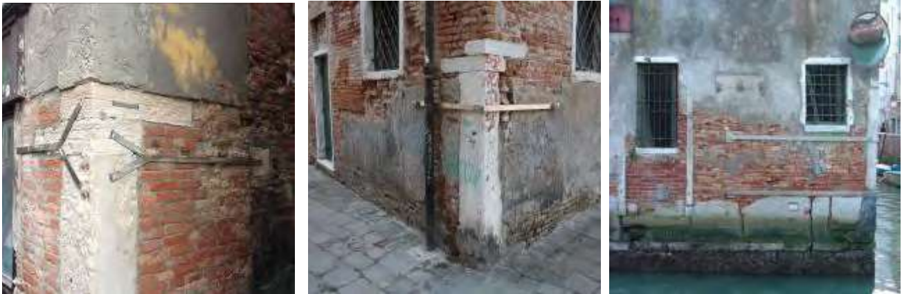
Figures 9-11 – Modern repairs using new materials and traditional systems
