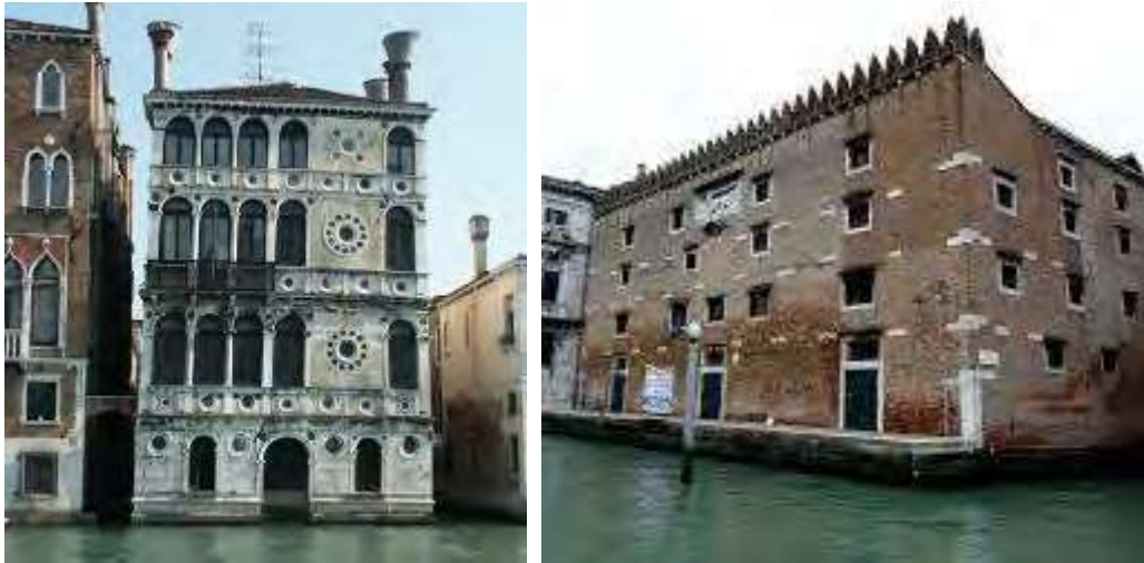
Figures 1-2 – Venice, Ca’ Dario, whose irregular geometry is partially intentional and partially due to structural damages. On the right: lines of fiube , along the façade of Fondaco del Megio
