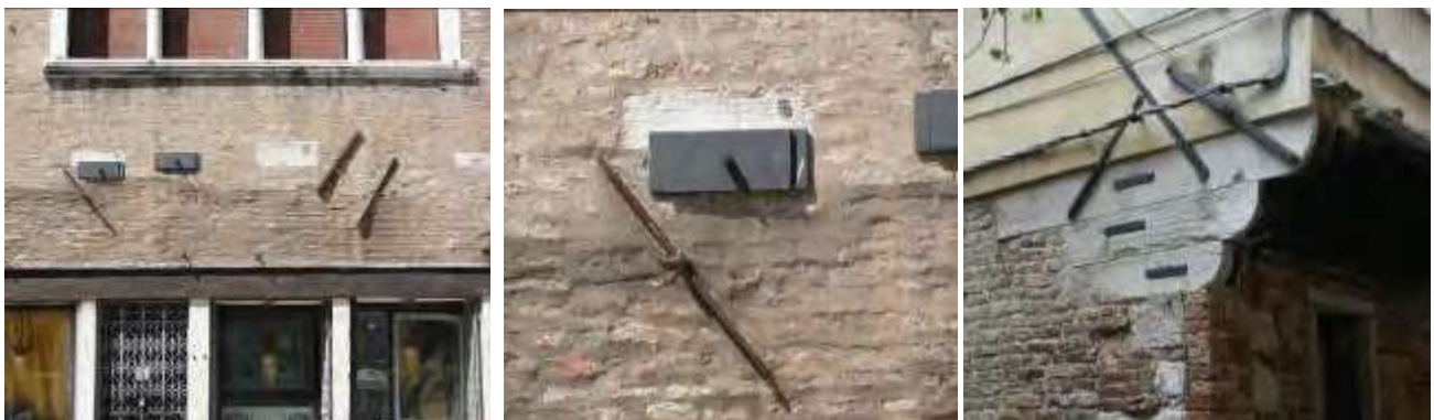
Figures 6-8 – Stratified connections of different periods in a medieval building and (on the right) in a “barbacane” (stone-and wooden shelves)
