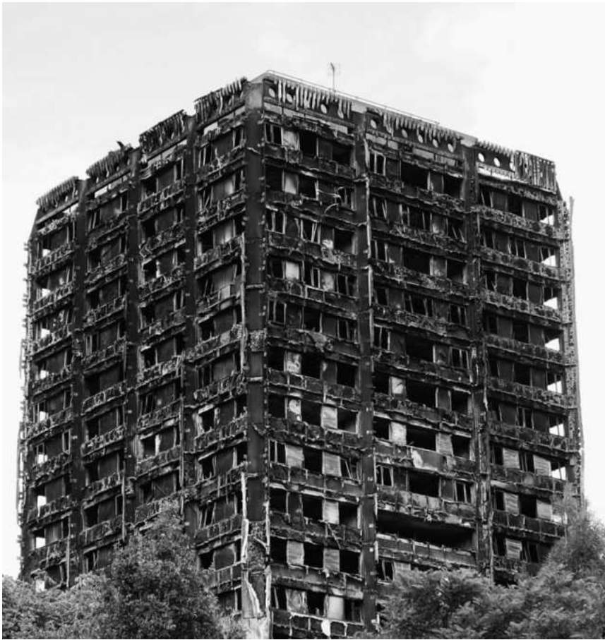
Figure 1.2: Grenfell Tower, London
