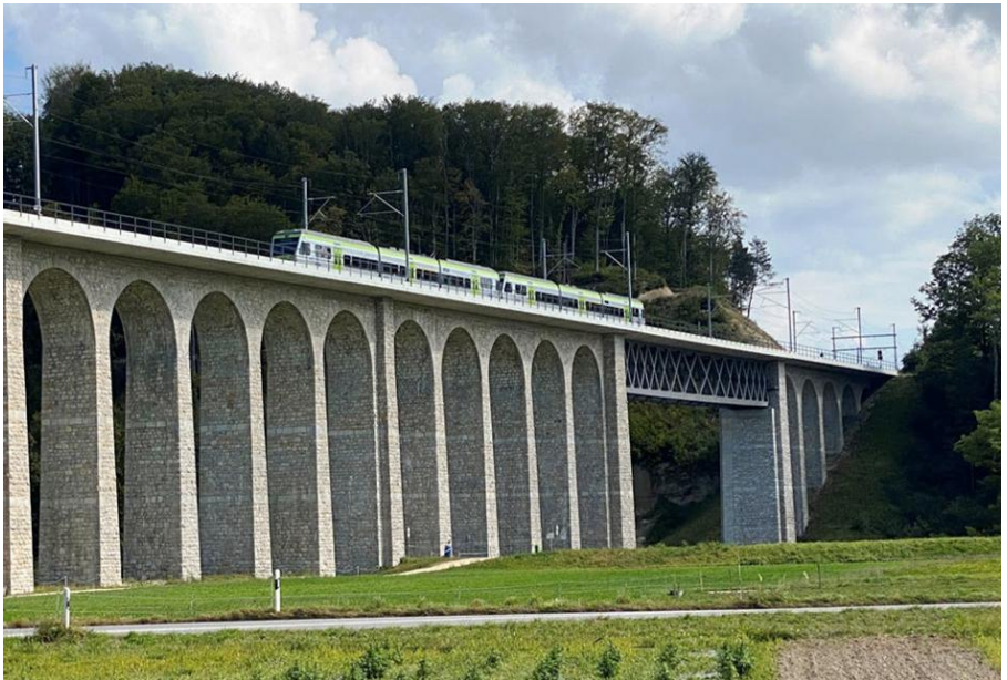
BLS Railway Viaduct over the Saane River near Gümmenen, Switzerland: modification of a heritage structure, originally built in 1901, from a single-track structure to a double-track structure by placing a wide reinforced concrete slab on top of the masonry structure in 2020
