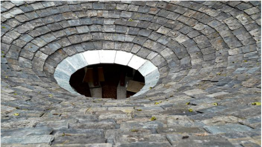
First build Form in 2019 by Students. First Site / First Form. The deconstruction and rebuild is planned for Fall 2023
