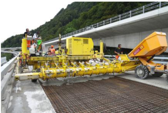
This 2.1-kilometer-long highway viaduct, built in 1969, was rehabilitated and strengthened in 2014–15 by means of the new UHPFRC (Ultra-High Performance Fiber-Reinforced Cementitious composite material) Technology (developed at EPFL). The realized project was cost-effective and did not impair the appearance of the viaduct which is a monument of national value. Photograph by the author
