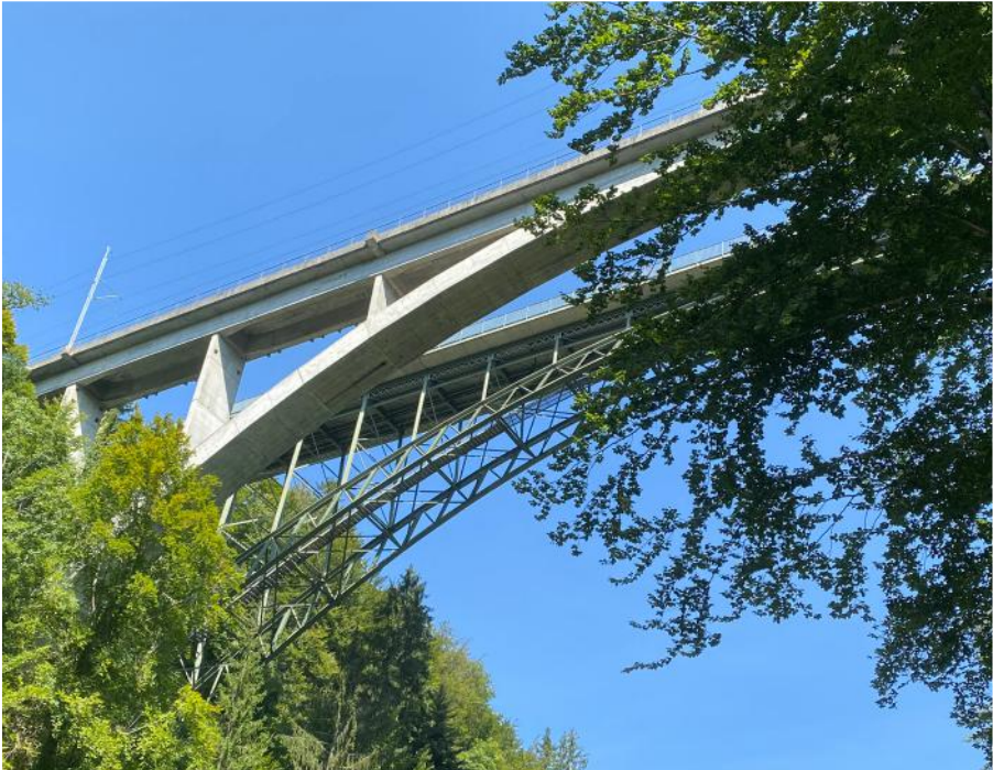
Engineering the existing means understanding construction methods and materials from different times, by means of the same arch structure typology: (1) lightweight riveted steel structure from the nineteenth century with a modified wider deck slab to accommodate modern road traffic needs, and (2) massive reinforced concrete structure from the 1970s in continued use to carry today's and tomorrow's trains. Photograph by the author
