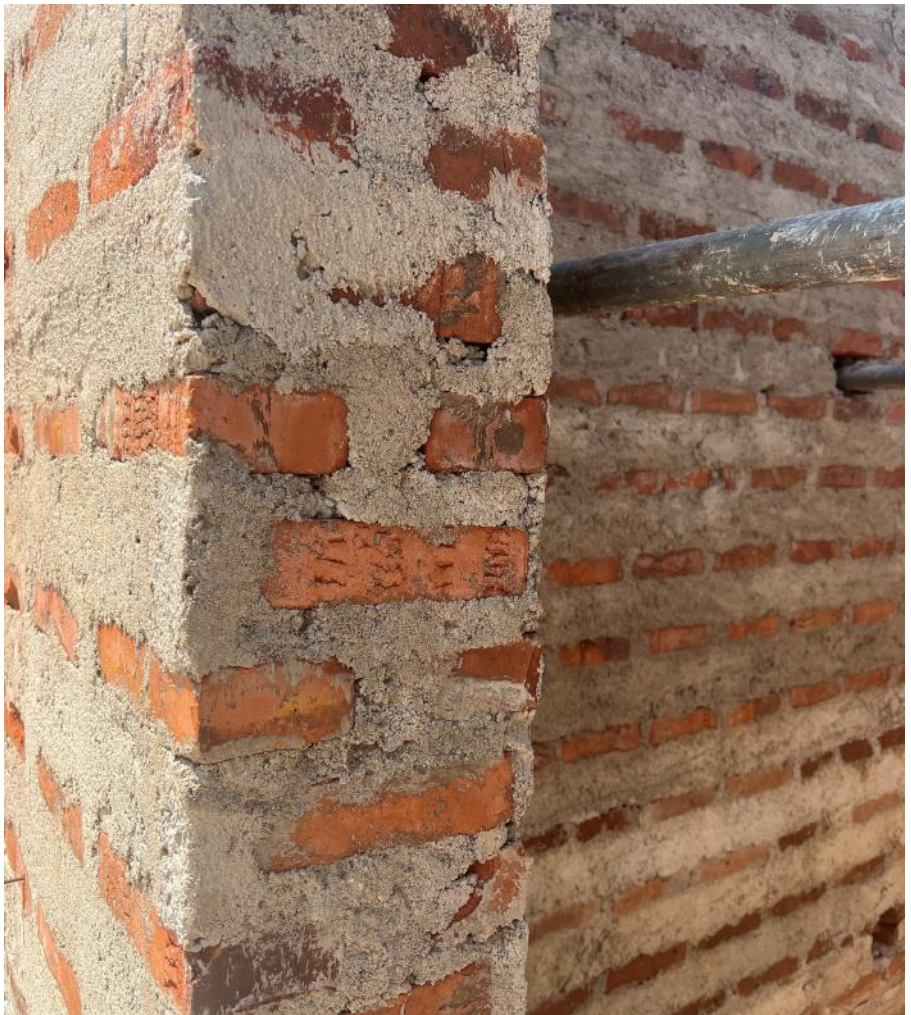
A construction site in Sri-Lanka, 2024, somewhere by the sea. Photographer: Jo Taillieu Architecten
