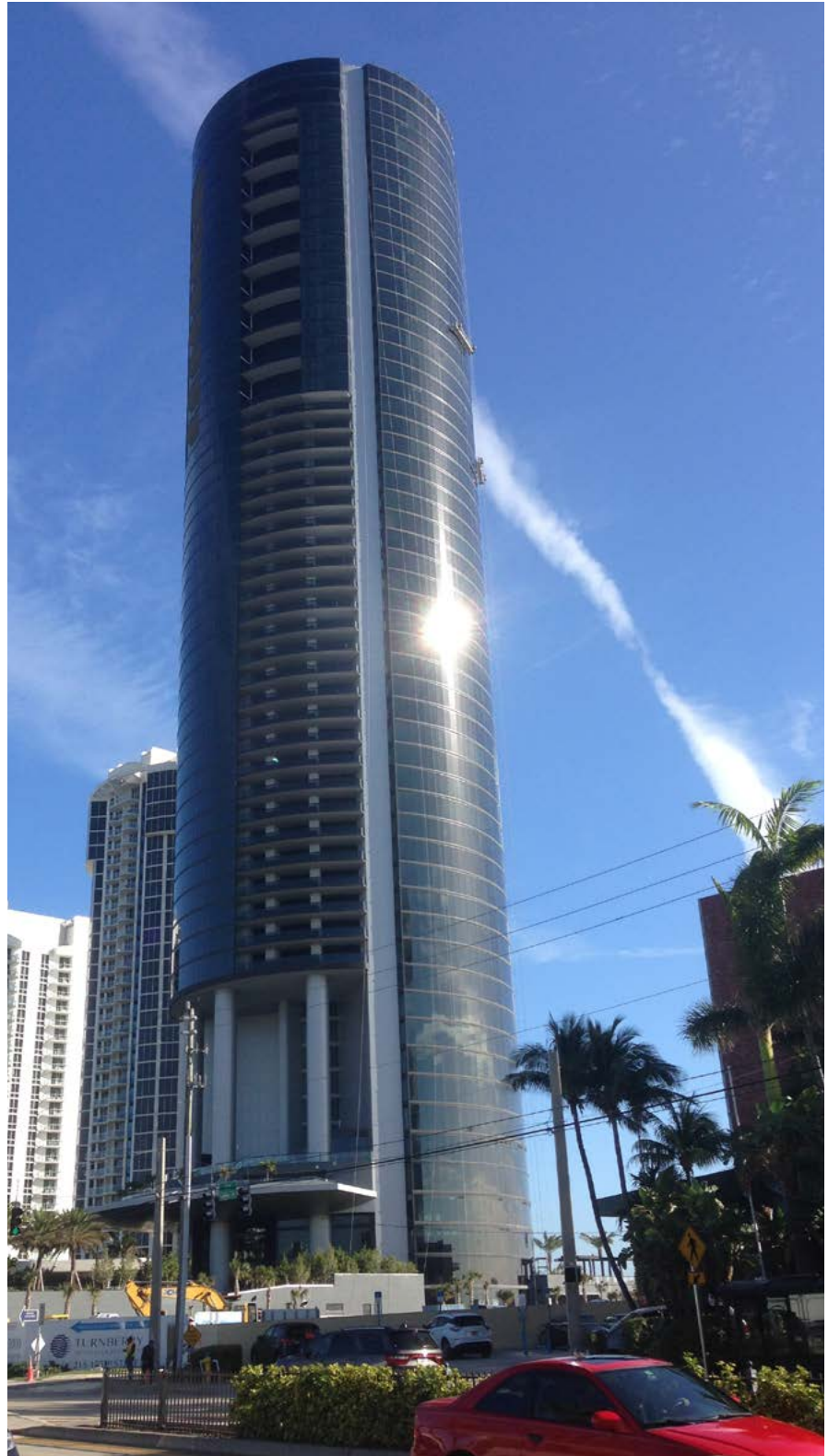
▲ Figure 14 –Porsche Design Tower, Miami (2017) extensively uses ionoplast interlayers in its façade
