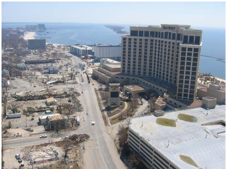
▲ Figure 17 – Biloxi. Despite the apparent integrity of the building envelope of MGM Mirage's Beau Rivage Hotel and Casino, after Hurricane Katrina there were many extensive damages.
