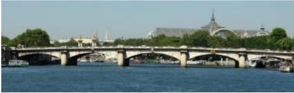
Fig. 2.36 Concordia bridge, Paris, France.
