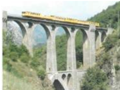
Fig. 2.40 Sejourne, Fontpederuse railway viaduct, France.
