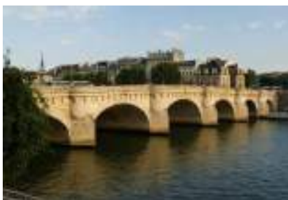
Fig. 2.33 Neuf bridge, Paris, France.
