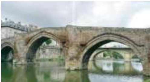
Fig. 2.18 Espalion bridge, France.
