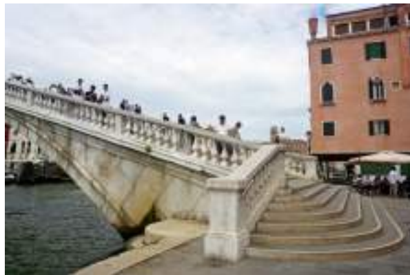
Fig. 3.21: Particular of the lateral parapets in Istria where the pipes are located in “Scalzi” bridge
