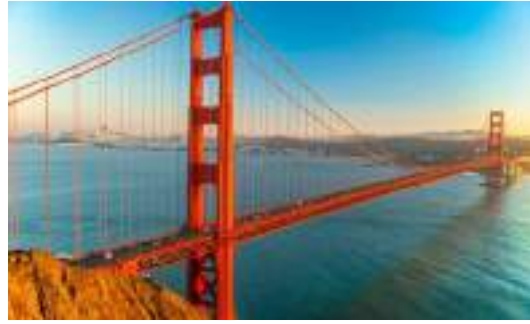
Fig. 2.2 Golden Gate bridge in S.Francisco, California
