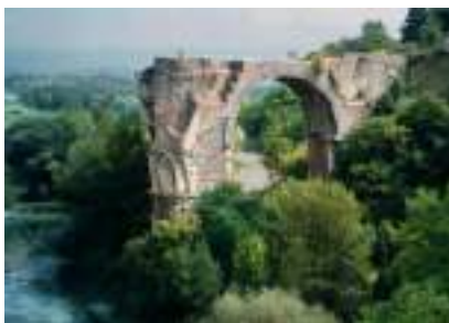
Fig. 2.3 Narni bridge, Italy.
