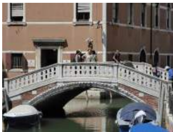
Fig. 3.18: "Frari" bridge. Railings made of Istria stone parapets
