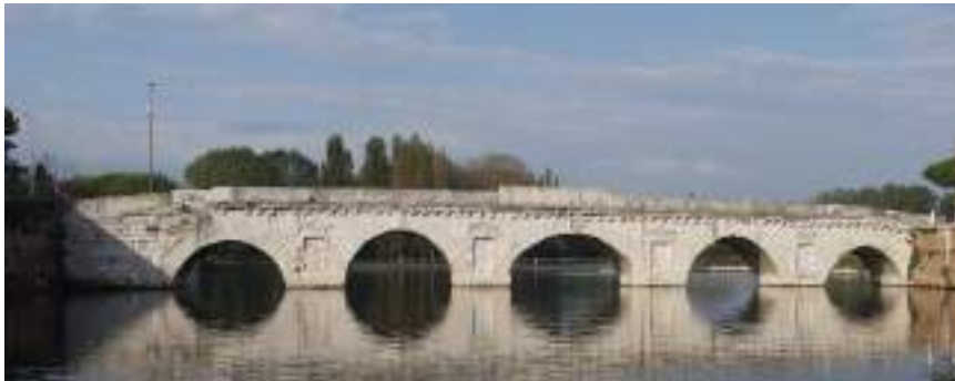
Fig. 2.15 Augusto bridge, Rimini, Italy.
