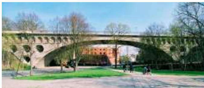
Fig. 2.4 Plauen bridge, Germany
