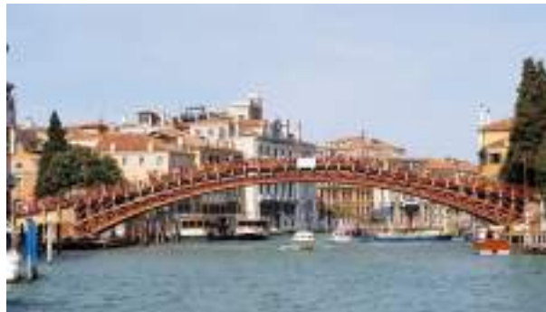
Fig. 3.4: : “De l'Accademia” bridge made of wood
