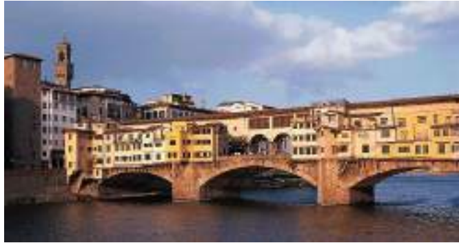
Fig. 2.20 Ponte Vecchio bridge, Florence, Italy.
