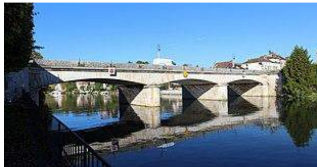
Fig. 2.37 Nemours bridge, Paris, France.
