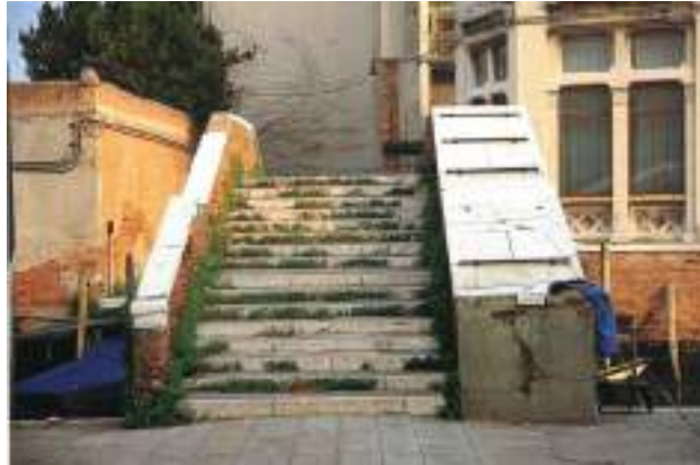
Fig. 3.20: Particular of the lateral structure realized in “De le Scuole” bridge
