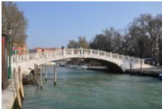
Fig. 3.7: "Prefetto" bridge. The vault is made by reinforced concrete
