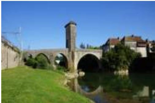
Fig. 2.24 Orthez bridge, France.
