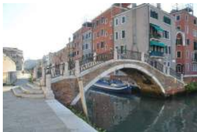
Fig. 3.16: Railings made of wrought iron supported by pillars in Istria stone of "De L'Arzere" bridge.
