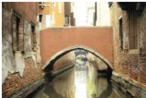
Fig. 3.8: "S.Rocco" bridge characterized by Hump (donkey-back) vault shape
