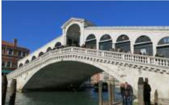
Fig. 3.5: "Rialto" bridge. The vault is made by Istria stone
