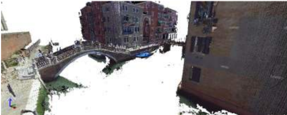
Fig. 7.2: "De L'Arzere bridge" Points cloud
