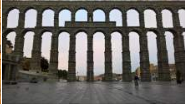
Fig. 2.10 Aqueduct of Segovia, Spain.
