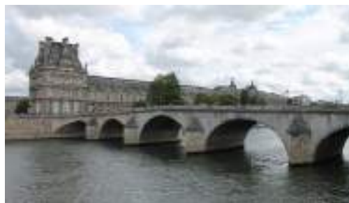
Fig. 2.34 Royal bridge, Paris, France.
