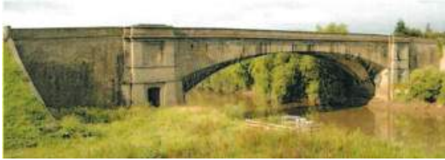
Fig. 2.38 Telford's bridge, Gloucester, England.
