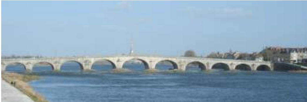
Fig. 2.35 Gabriel bridge, Blois, France.
