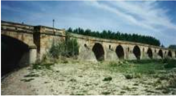
Fig. 2.13 Andùjar bridge, Andalusia, Spain.
