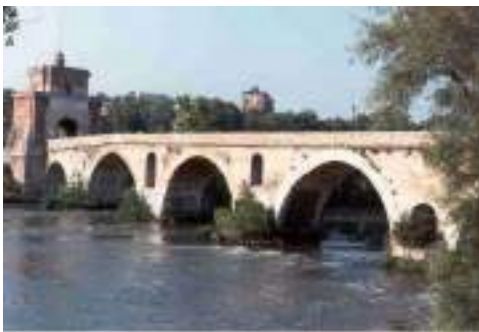
Fig. 2.11 Milvio bridge, Rome, Italy.
