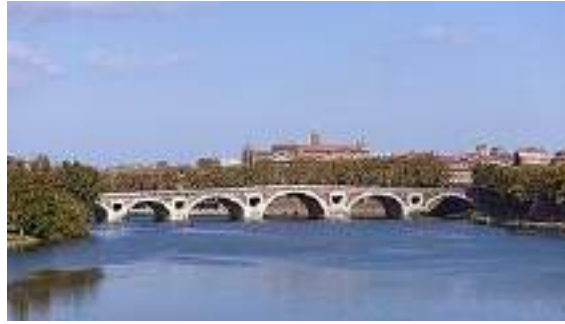
Fig. 2.28 Ponte Amidonniers, Tolosa, Spain.
