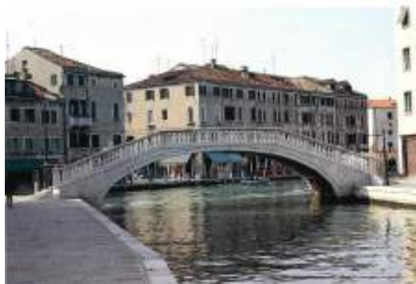
Fig. 3.11: "De la Ceraria" bridge, located in Rio Novo, characterized by polycentric vault shape, designed by Miozzi in 1932.
