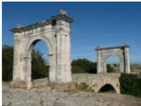
Fig. 2.16: The Flaviano Bridge, Saint-Chamas, France.
