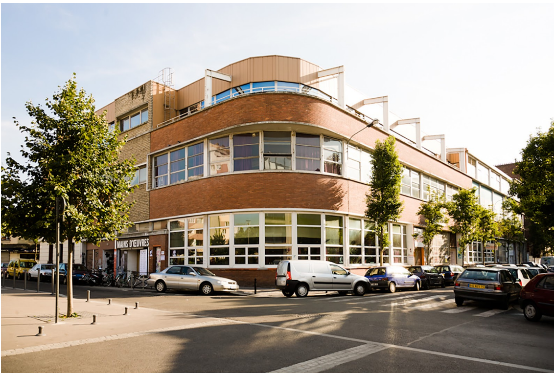
Figure 4.16 - Exterior of Mains D'œuvres. Author: Vinciane Verguethen
