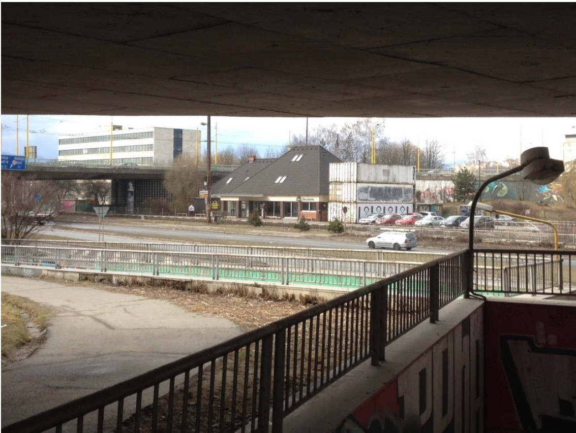
Figure 4.5 - Exterior view of Stanica Žilina-Zaricie in 2018 - Author: Francesco Campagnari
